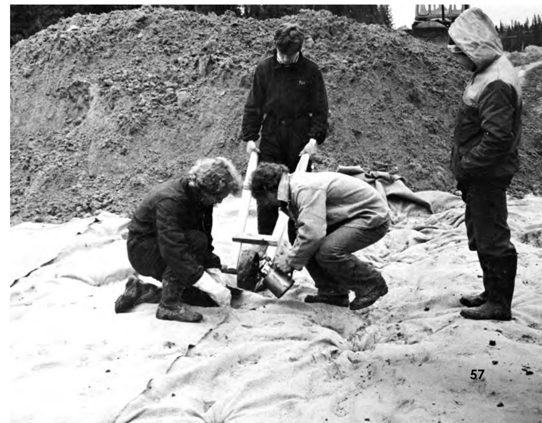
Forestry Faculty Students during practical training at the All-Union production enterprise «Komilesprom» laid a geofabric roadbed on a swampy stretch of Nizhny Odes - Vuktyl road. 1982
