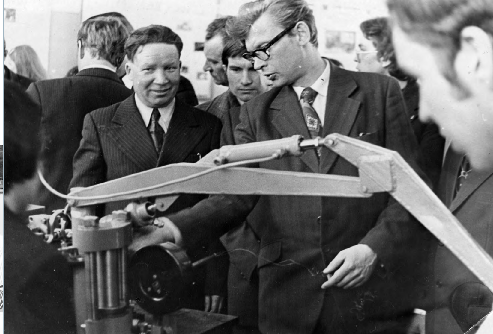
Forest Technology Faculty Associate Professor, G. P. Drozdovskiy, demonstrates the hydraulic manipulator model. 1978
