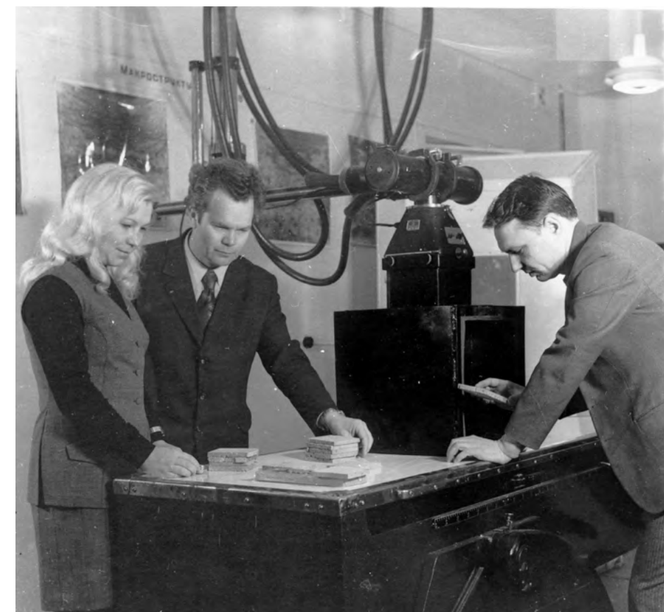
| Rock analysis on an X-ray machine. 1974.
